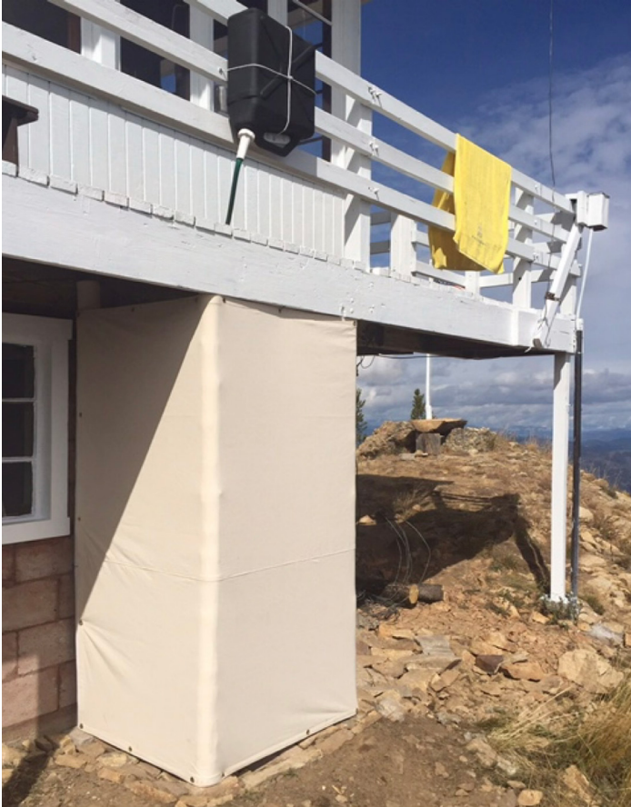
Fig. 18-19 Showers at Bear Mountain and Hells Half. The most efficient solar shower we've used was a design I found in Mother Earth News. It involved a truck inner tube, hose, coupling, and garden sprayer. Photo by Rhett Moak (fig. 18).
